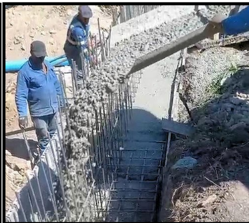
Casting the concrete for the spillway.
