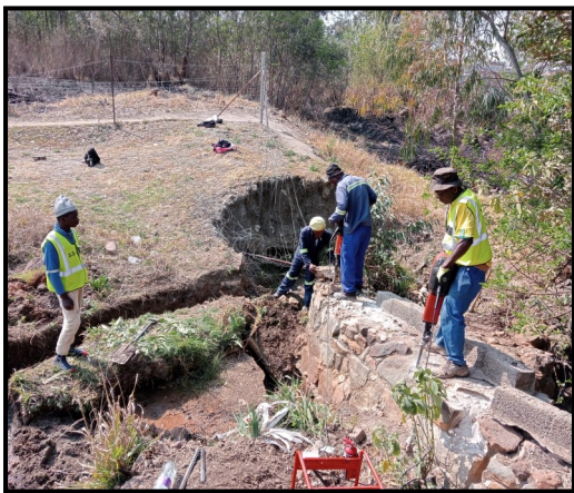
Collapsed wall being broken down.
