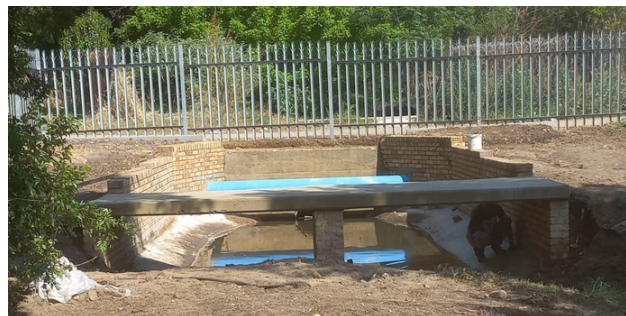
Litter trap construction completed
